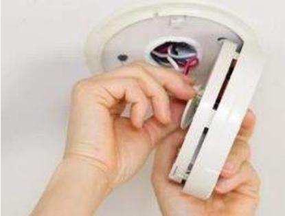
A person's hands are shown removing the cover of a smoke detector, revealing the internal wiring and components. |
